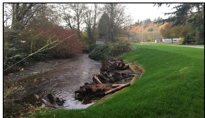
Restored stream bank with added wood to prevent future erosion
