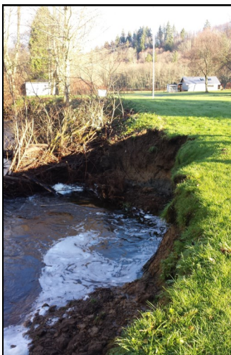
Bankside erosion resulting in the loss of property
