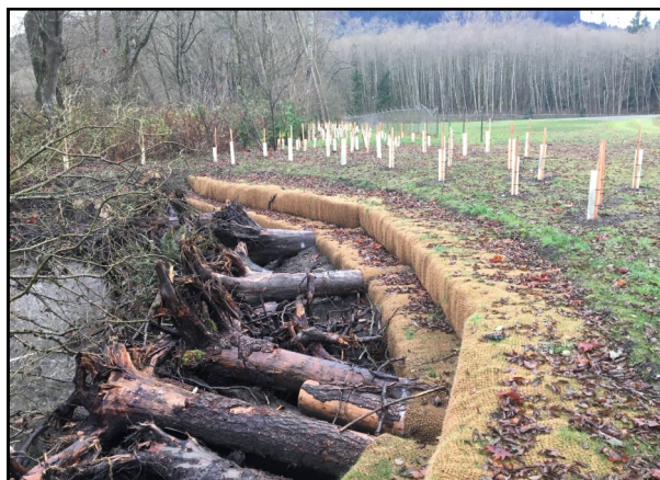
Completed Restoration Site with Large Woody Debris (LWD)
